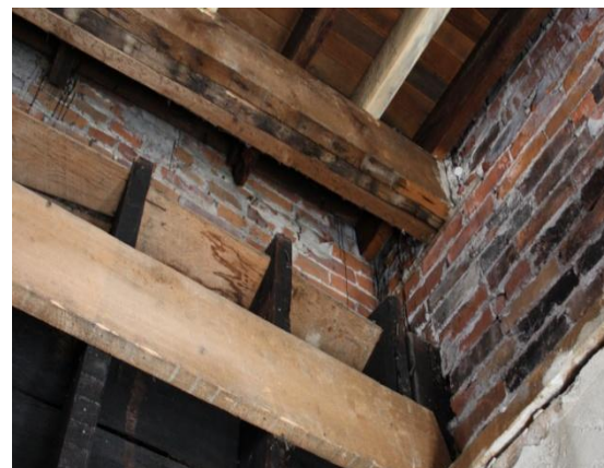
Interior View, 3 rd Floor, Queen's Hotel
